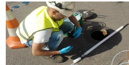
Installation and sampling
